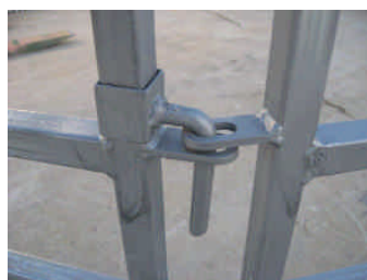
PANEL SLIDING PIN LOCKING DEVICE
